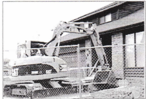
Crews began cleaning up Lynnview Ridge in the summer. (CBC)
